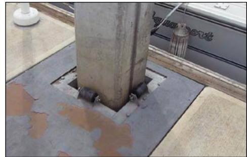
square concrete guide pile
