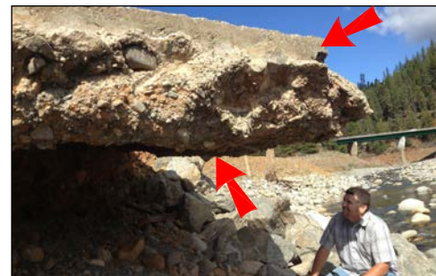
flood water undercut launching ramp
