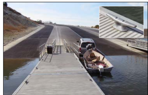
minimum of 5 ft clear between edge hardware
