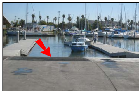
vertical curve at head-of-ramp
