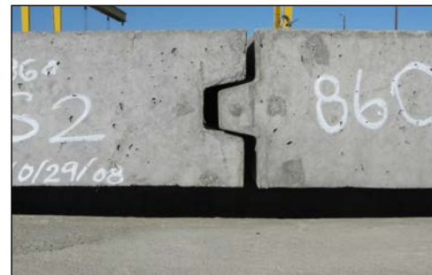
precast concrete panel keys
