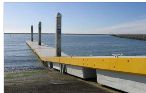
non-articulated float section at far end
