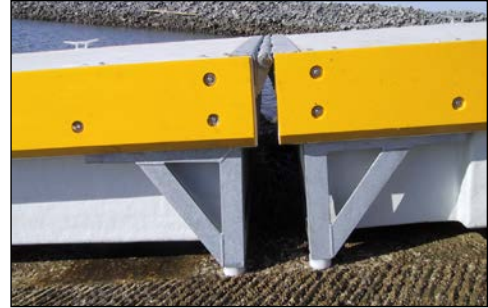
unnneeded downslope support leg(s)
