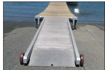
leading edge of gangplank
