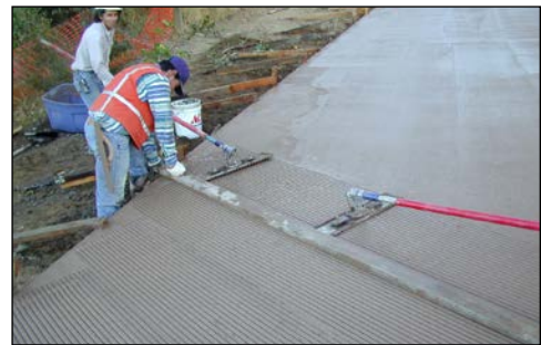
creating diagonal V-grooves in wet concrete
