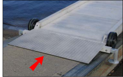
1/2 inch max gangplank leading edge
