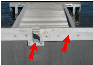
gangplank lifted up to see cable slot and wearstrip
