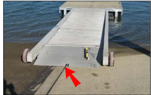
gangplank with centerline cable
