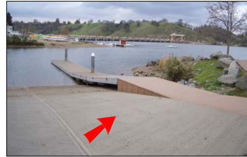
launching ramp apron merging with vertical curve
