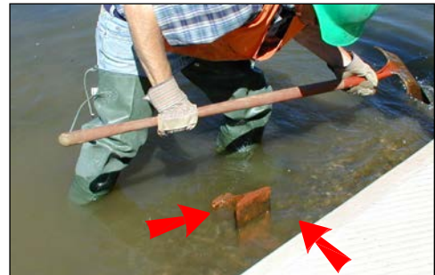
precast panel is nearing catch cleat as worker clears away plowed gravel
