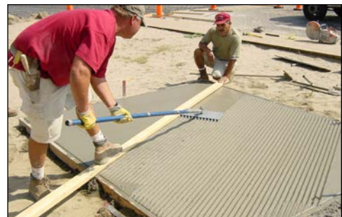
on site V-groove test panel
