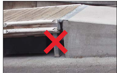
“no-no” float legs next to abutment
