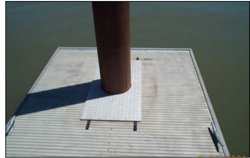
sliding pile yoke cover on round pile
